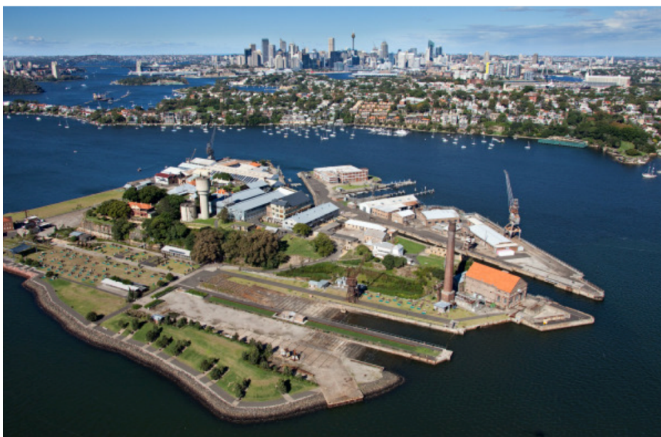
Fig 1 – Aerial photograph of Cockatoo Island as it is today. Image by Sydney Harbour Federation Trust.
